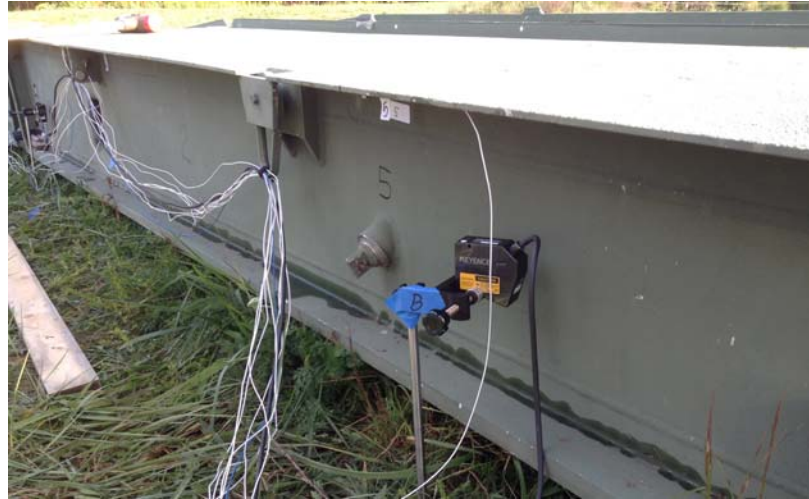
(b) Sensor close-up on REB top flange
